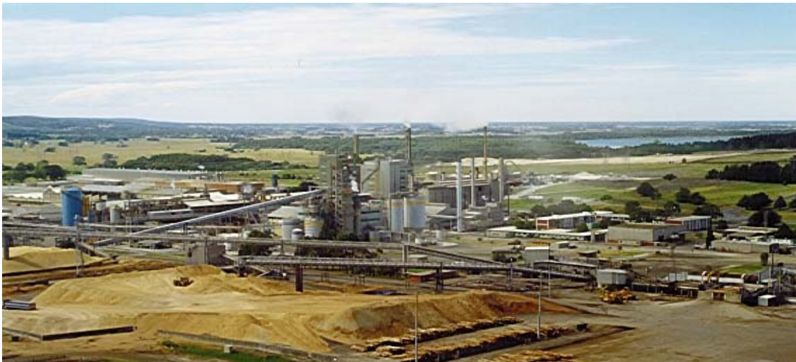
Photo courtesy of Maryvale Mill
