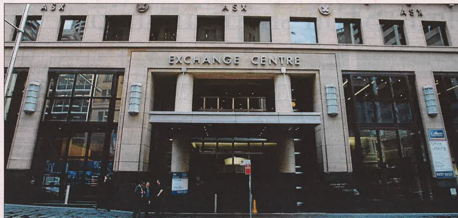
Exchange Centre in Sydney's Bridge Street, which houses the Australian Securities Exchange, is open to bids again.
